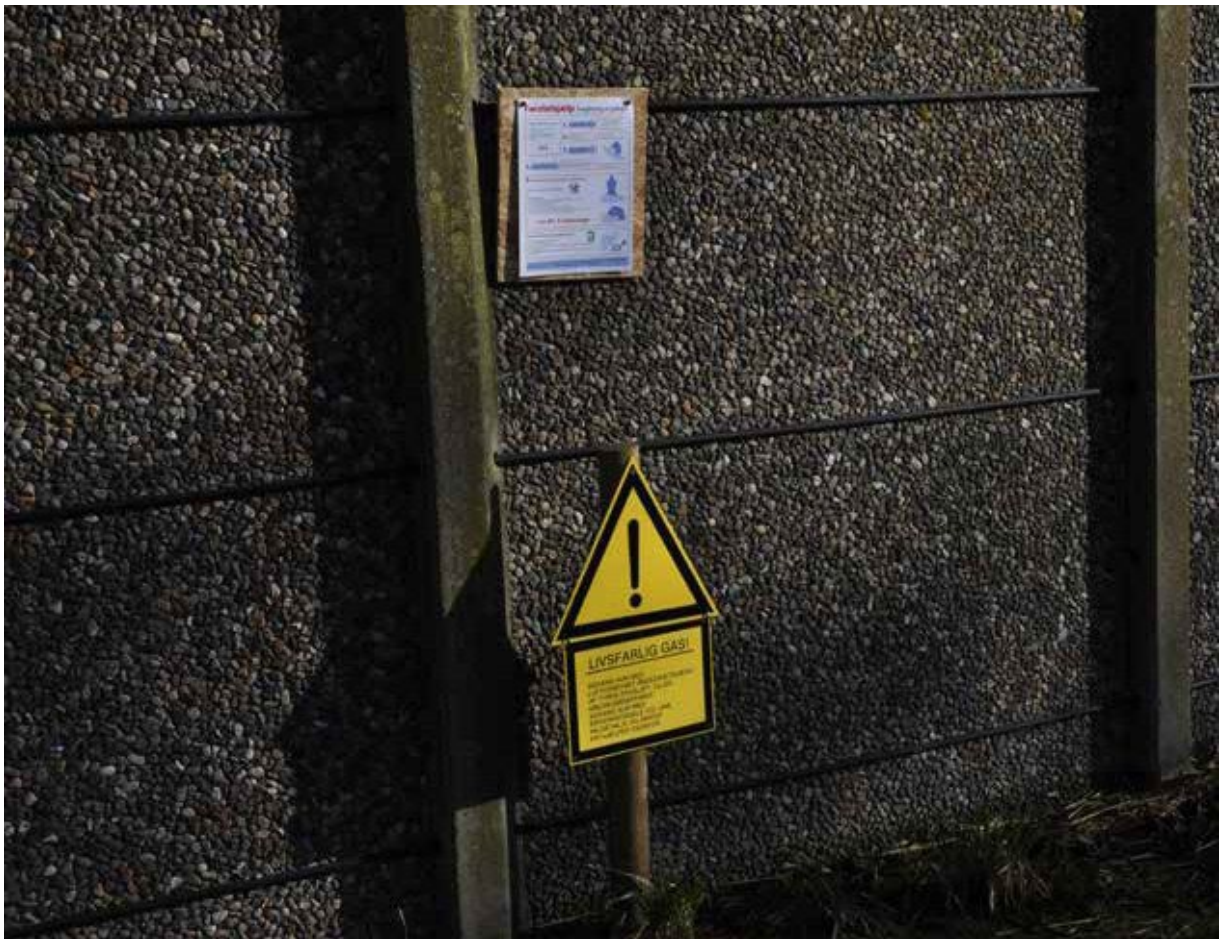
Proper signage at a slurry tank, including poison hazard and poison first aid warning signs.
