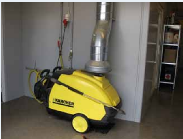
Stationary compressors should be placed in a sound proofed room with an air exhauster. This causes less noise.
